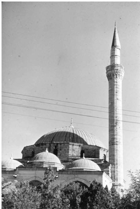
Figure 2.40 The spire of the Mustapa Paša jamija (mosque), built c. 1493, after the earthquake of July 1963 in Skopje. Its tip was knocked so far sideways that the minaret seems to defy the laws of equilibrium. In spite of the violence of the earthquake, there was no structural damage.
