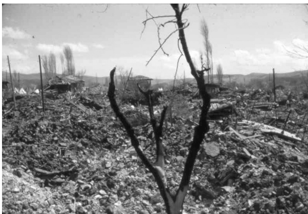
Figure 2.68 The ruins of a village in the Gediz area, almost entirely of timber-framed houses, which survived the earthquake of 28 March 1970 with reparable damage, but was burnt down by fires started by the shocks.
