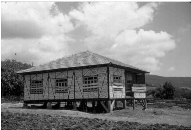
Figure 2.67 Another low-vulnerability traditional timber-framed house in the Gediz area, of a type too expensive to build in the reconstruction of the rural areas.
