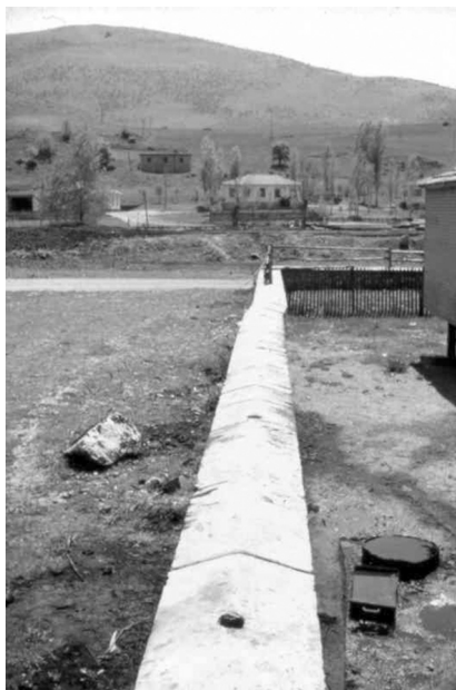
Figure 2.33 A masonry fence wall, built in 1957, straddling the North Anatolian fault zone at İsmet Paşa railway station, displaced by creep movements associated with the earthquake of 1951.
