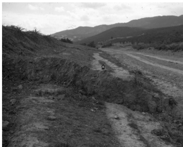
Figure 2.35 A dirt road that crosses the fault break caused by the earthquake of 28 March 1970 in Turkey was repaired a few days after the event. The rut on the repaired road was made by the passage of wheeled carts after heavy rains that followed the event. The figure shows the rut offset after its formation.
