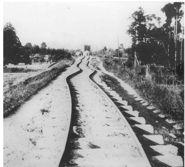
Figure 2.88 Permanent ground deformation associated with the Mino Owori earthquake of 28 October 1891 in Japan (Milne et al. 1892).
