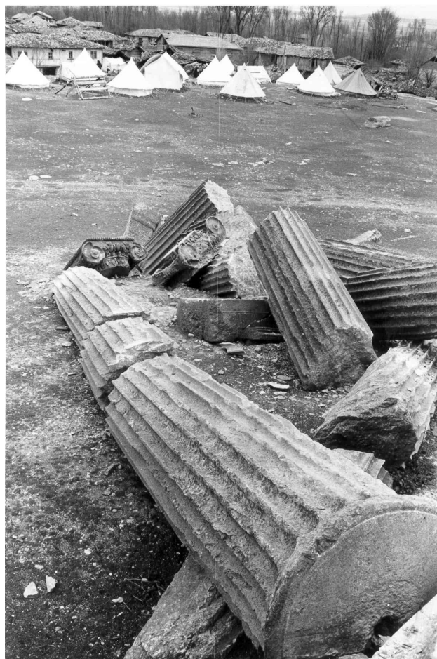
Figure 2.48 Two of the three columns of the Roman temple of Zeus at Aizani which had been repaired well before the earthquake, shown on the right in Figure 2.45, after their collapse in the Gediz earthquake of 28 March 1970. In the background is the village of Çavdahisar, which was badly damaged.
