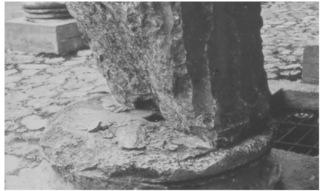
Figure 2.46 Characteristic damage to one of the columns of the temple of Zeus at Aizani caused by the deliberate hewing off of its base drum, probably for the lead of its dowel.
