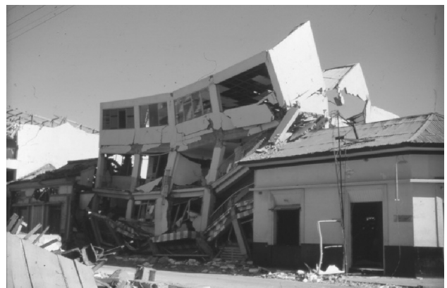
Figure 2.71 Contrasted response to the Managua earthquake of 23 December 1972 of two contiguous structures of different materials and methods of construction. An engineered, but badly built, reinforced-concrete four-storey building collapsed completely, while the adjacent one-storey house, built with traditional wood and pumice-block materials ( takazal ) with a light tin roof, suffered no serious damage.
