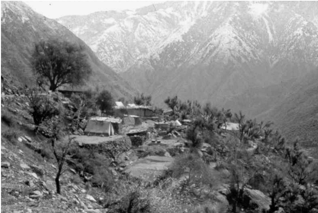
Figure 2.81 A close-up view of a settlement perched on the right bank of the Indus gorge (on the Hazara side) further to the north of that shown in Figure 2.80. All houses made of stone without reinforcing wooden beams were damaged beyond repair and a few were carried away by small local slides.
