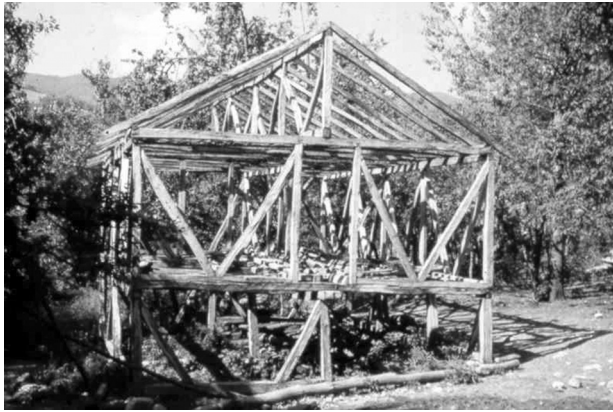
Figure 2.66 One of the few timber-framed houses under construction after the Mudurnu earthquake in Turkey, of a traditional type that replaced the more fashionable, but vulnerable, unreinforced hollow-brick and low-quality reinforced-concrete houses.
