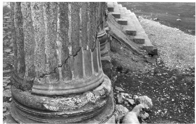
Figure 2.47 Detached corner repair with cement at the base of one of the columns carried out before the Gediz earthquake of 28 March 1970.
