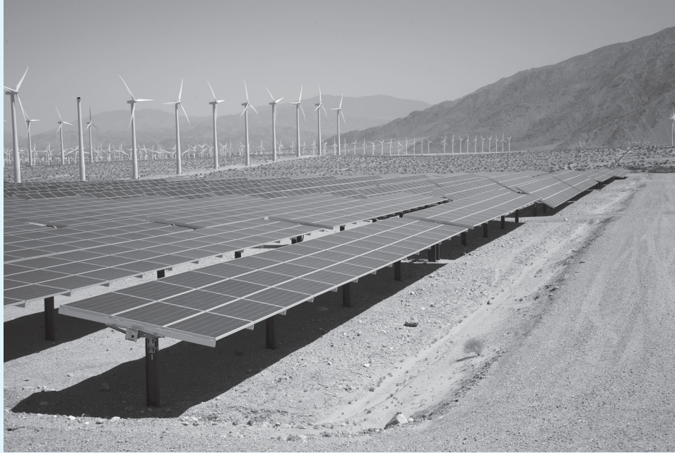
FIGURE 1.1 South Africa's Jasper Solar Farm
