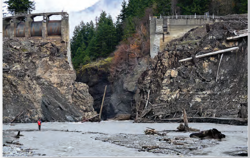
▲Figure 1.1 Dam removal for river restoration. Removal of Glines Canyon Dam on the Elwha River, Washington, began in November 2012 to restore river ecosystems. [Brian Cluer/NOAA.]
