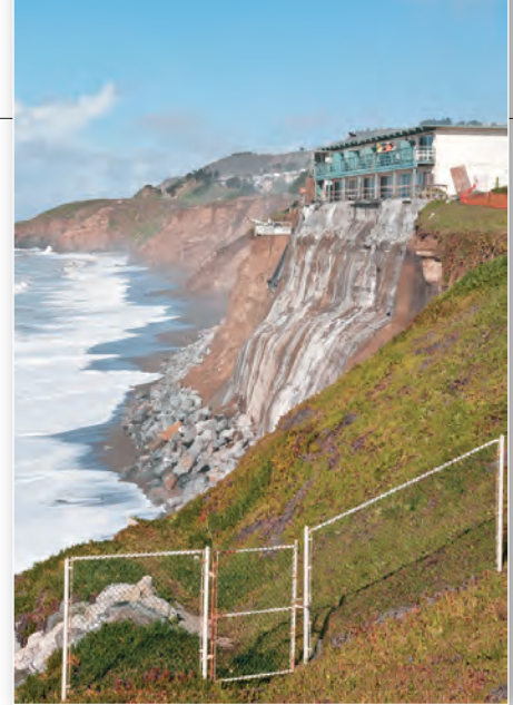
(c) Wave action and heavy rainfall caused slope instability along the Pacific Coast of south of San Francisco in January 2010. When a threshold was reached, the bluffs collapsed and the cliff face retreated inland some 30.5 m (100 ft).
