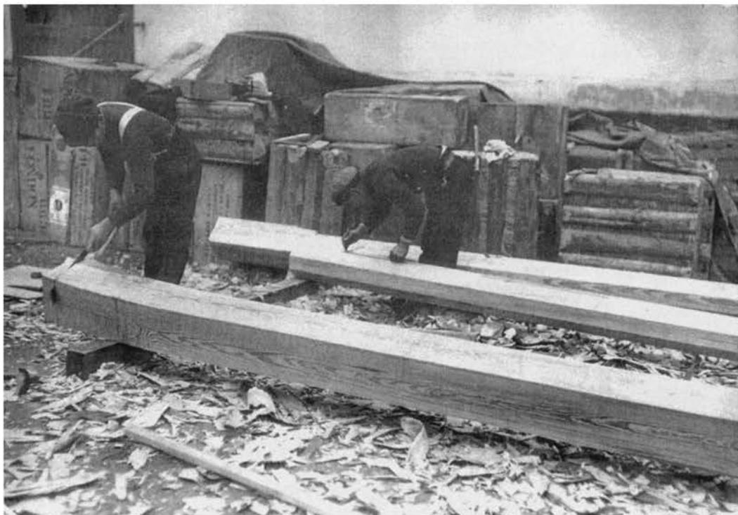
Figure 6. Japanese carpenters using traditional tools and techniques to prepare structural timbers for construction work at the 1910 Exhibition. Source: Private Collection
