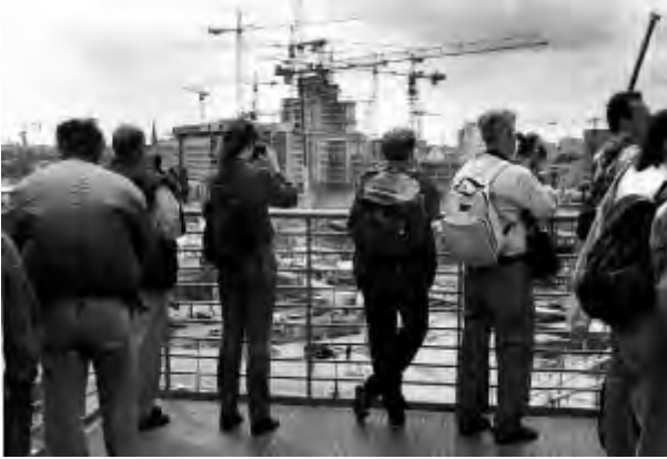
Figure 1.1. Watching the construction process at Potsdamer Platz from the viewing platform of the INFOBOX, Leipziger Platz (5 July 1996). (Source: Landesarchiv Berlin/Edmund Kasperski)
