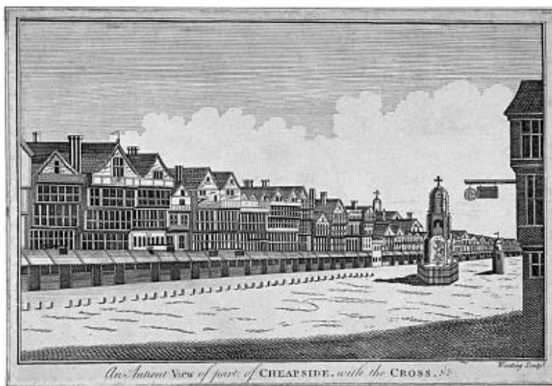
Figure 2.16 Cheapside, London, UK (1638) typifies the urban streetscape of the time with open fronted ground floor shops and living accommodation above. (Source: Guildhall Library)
