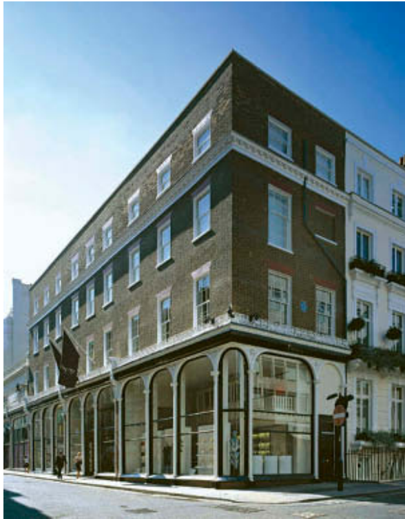
Figure 2.20 One of the first plate glass shopfronts in England installed at Asprey's, London, UK (c 1860). (Source: Arcaid/Richard Bryant )
