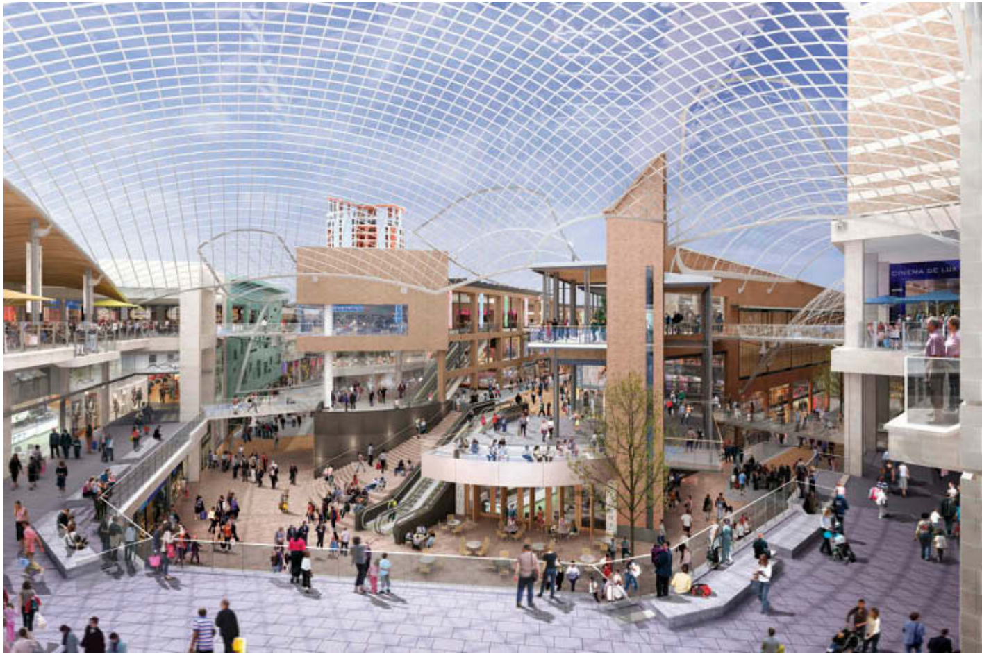
Figure 1.18 A glazed diagrid covers the naturally ventilated public space, to form the focus of the Bristol City Centre Expansion, Bristol, UK (2008). (Source: Chapman Taylor)
