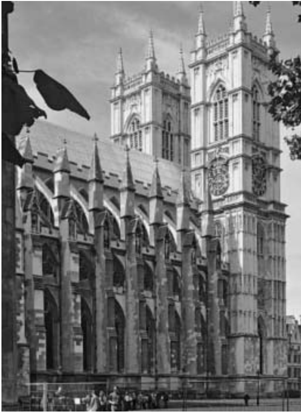
Figure 1.11 Westminster Abbey's 13 th -century nave, extended 'in keeping' from 1375 (by masons John Palterton and Henry Yevele) and western towers (completed in 1735–45 to designs by Thomas Hawksmoor)
