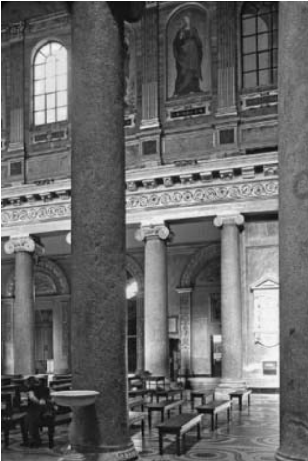
Figure 1.10 The nave arcade of the 12 th -century St Maria Trastevere, Rome, showing spolia from the Baths of Caracalla
