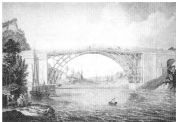
Fig. 1.1 Ironbridge, Coalbrookdale 1777–9 (engineer Abraham Darby).
