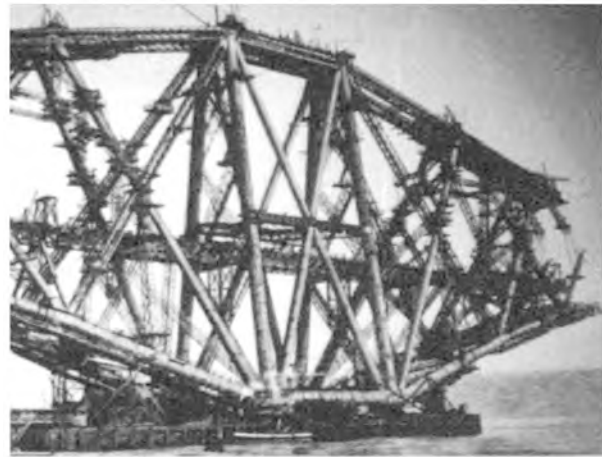
Fig. 1.5 Forth Railway Bridge under construction, late 1880s (engineer Benjamin Baker).
