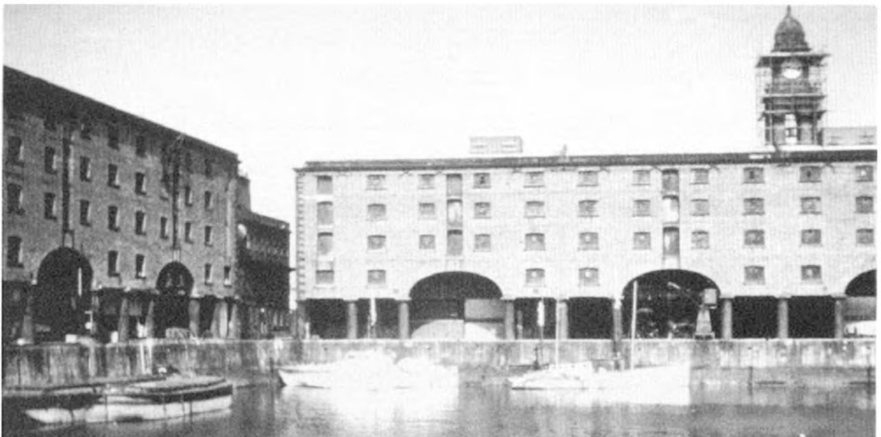
Fig. 11 Albert Dock, Liverpool 1848 (architect Philip Hardwick; engineer Jesse Hartley).
