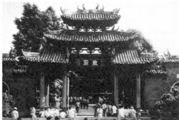
Fig. 2 Temple gateway, Canton (three tiers of beams).
