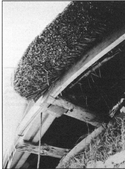
Fig. 2: Strawbale, roundwood timber and thatch. Ecological use of local and renewable materials in Ireland.
