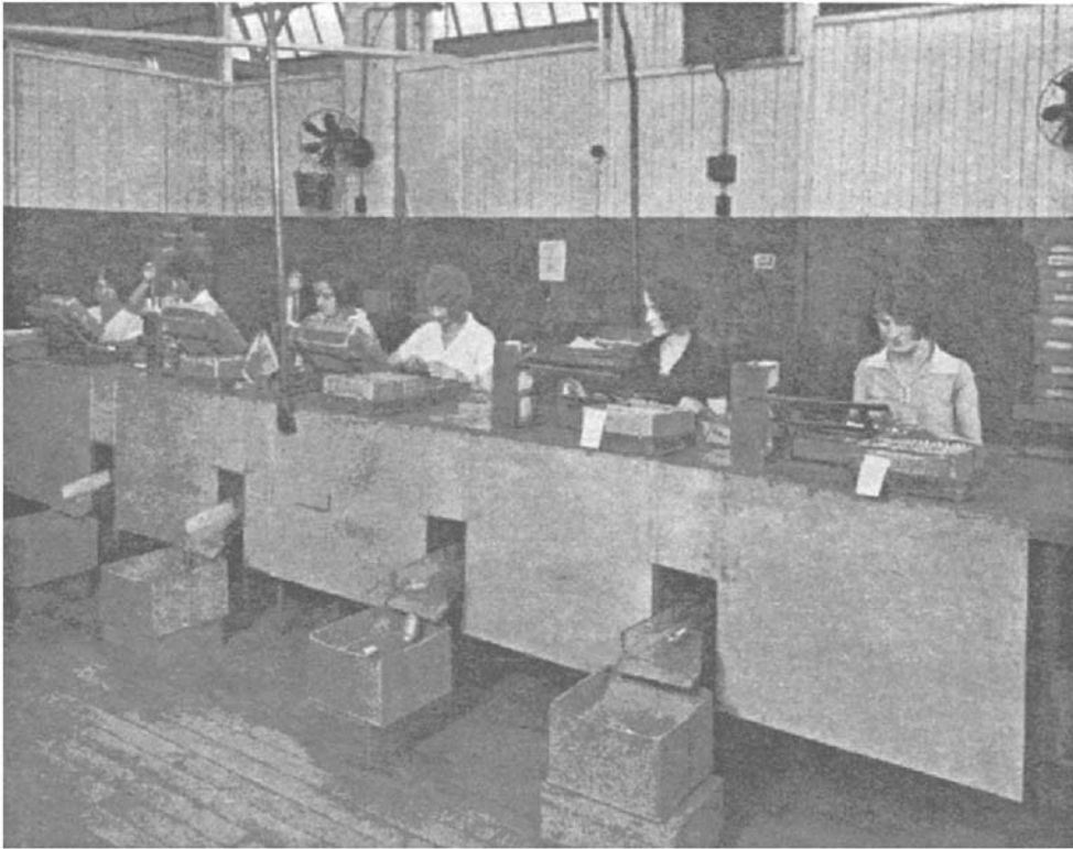
FIGURE 3 PHOTOGRAPH OF RELAY ASSEMBLY TEST ROOM
