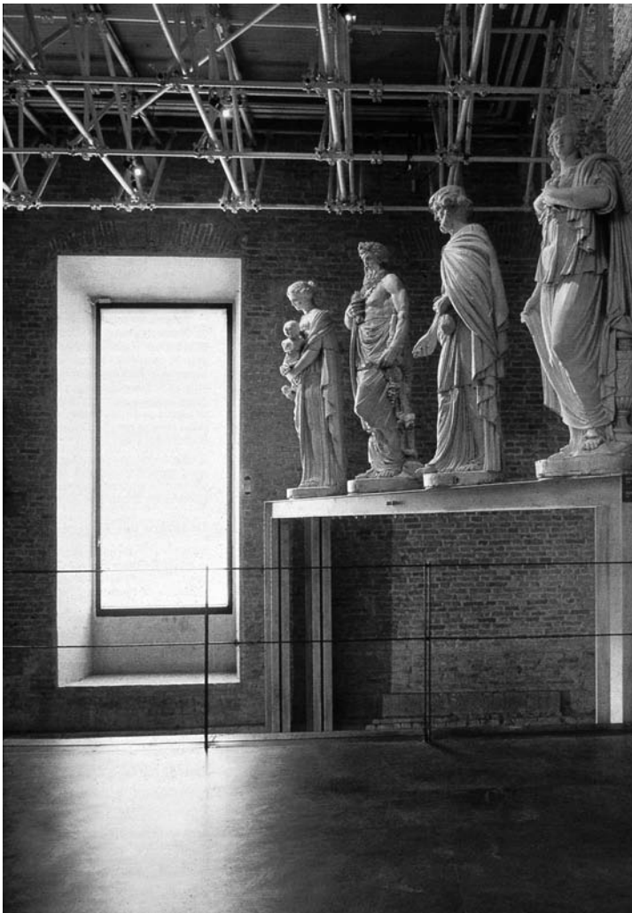
1.5 Heavy stone sculptures raised on a light structural frame. Architect Guido Canali: The National Gallery ('La Pilotta') (1986), Parma, Italy.
