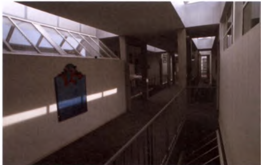
▷ Corridors of the Reiterstrasse Office building in Bern are lit with natural light, partly hidden from the field of vision, filtering between obstructions, leading to a low luminance level, glare-free, but pleasant space.
