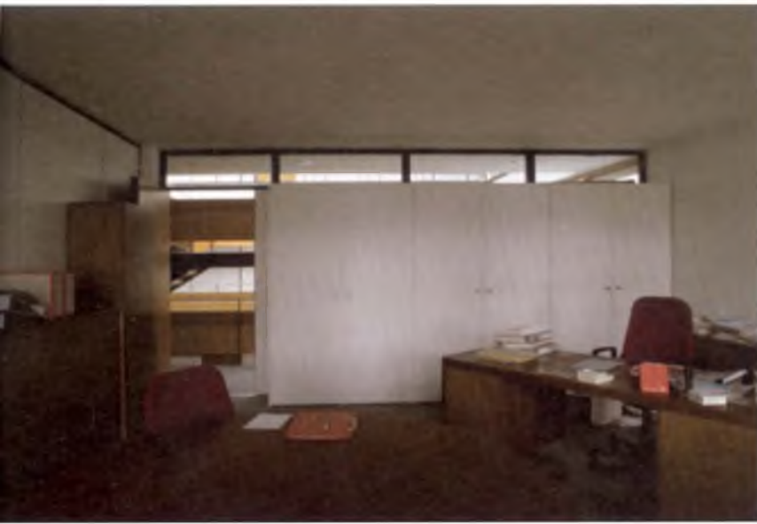
△ These secondary daylighting windows are clearly undersized with regard to their potential to add extra daylight to the corridors from the daylit offices.
