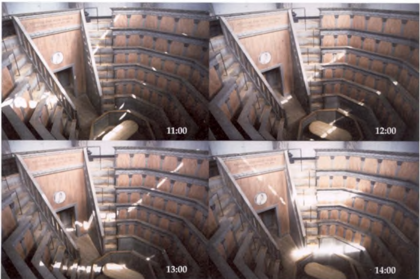
Δ Sequences of pictures of sunlight penetration at referenced dates such as solstices and equinoxes showing the response of the architecture or the daylighting system to incoming sunlight.
