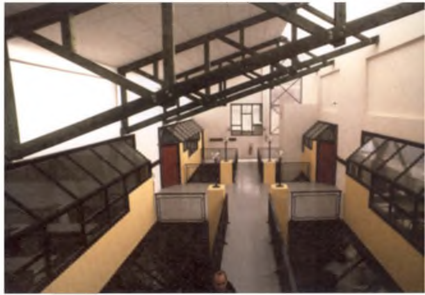
△ In Collège La Vanoise, Modane, France, the most attractive daylighting feature is the tilted secondary lighting system allowing daylight to penetrate from the atrium roof to the interior. The tilt angle of the windows leads to a transmitted light equal to 3 times that transmitted by vertical windows. Daylight distribution in classrooms becomes balanced and the general impression is of a very bright space.
