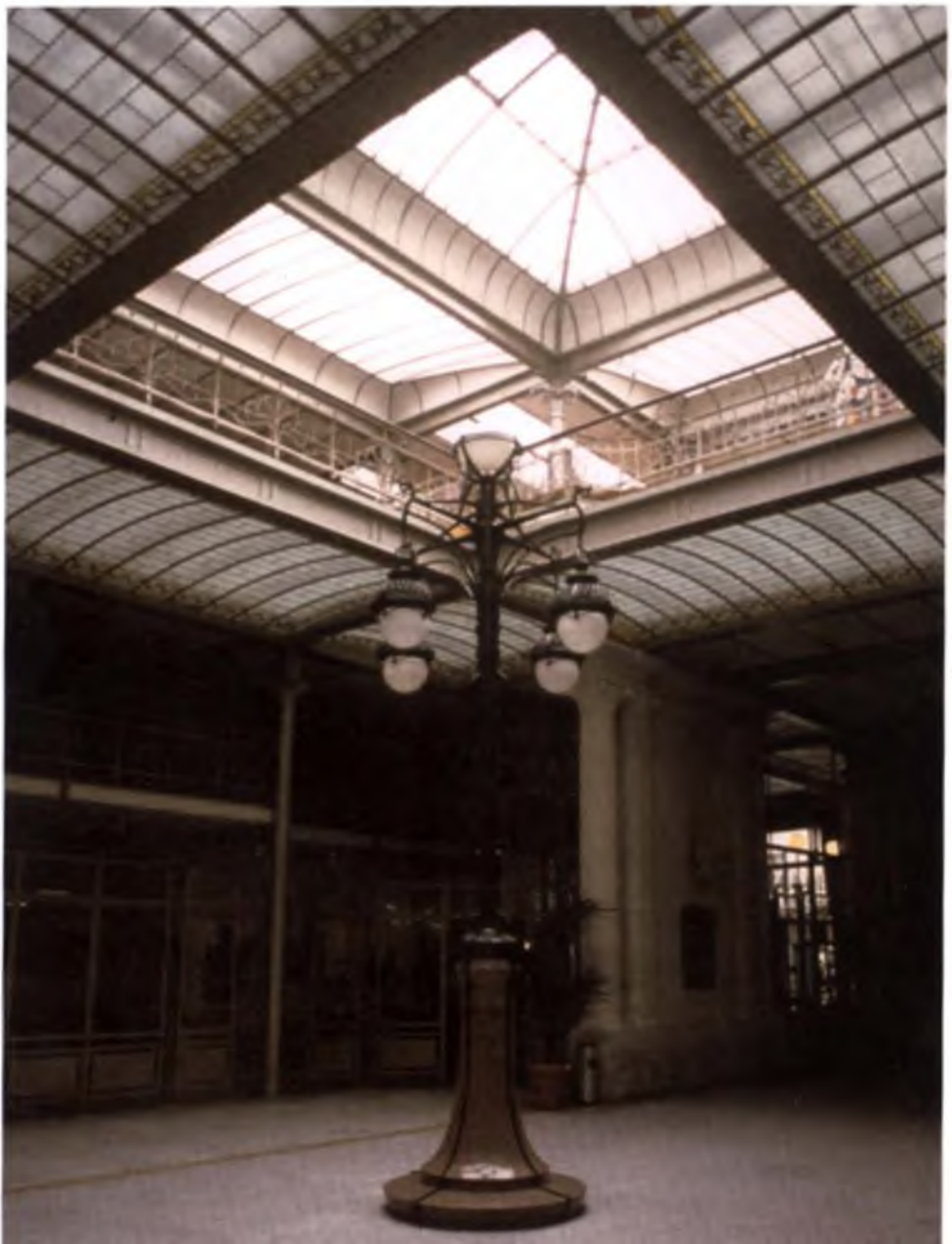
▷ The translucent floors and ceilings of the Waucquez Department Store in Brussels allow daylight to penetrate deep into the building, because their area (comparable to the area of the glazed roof) compensates for the optical losses associated with the triple absorption of light coming from the outside. At ground level, daylight factors reach values above 1%.
