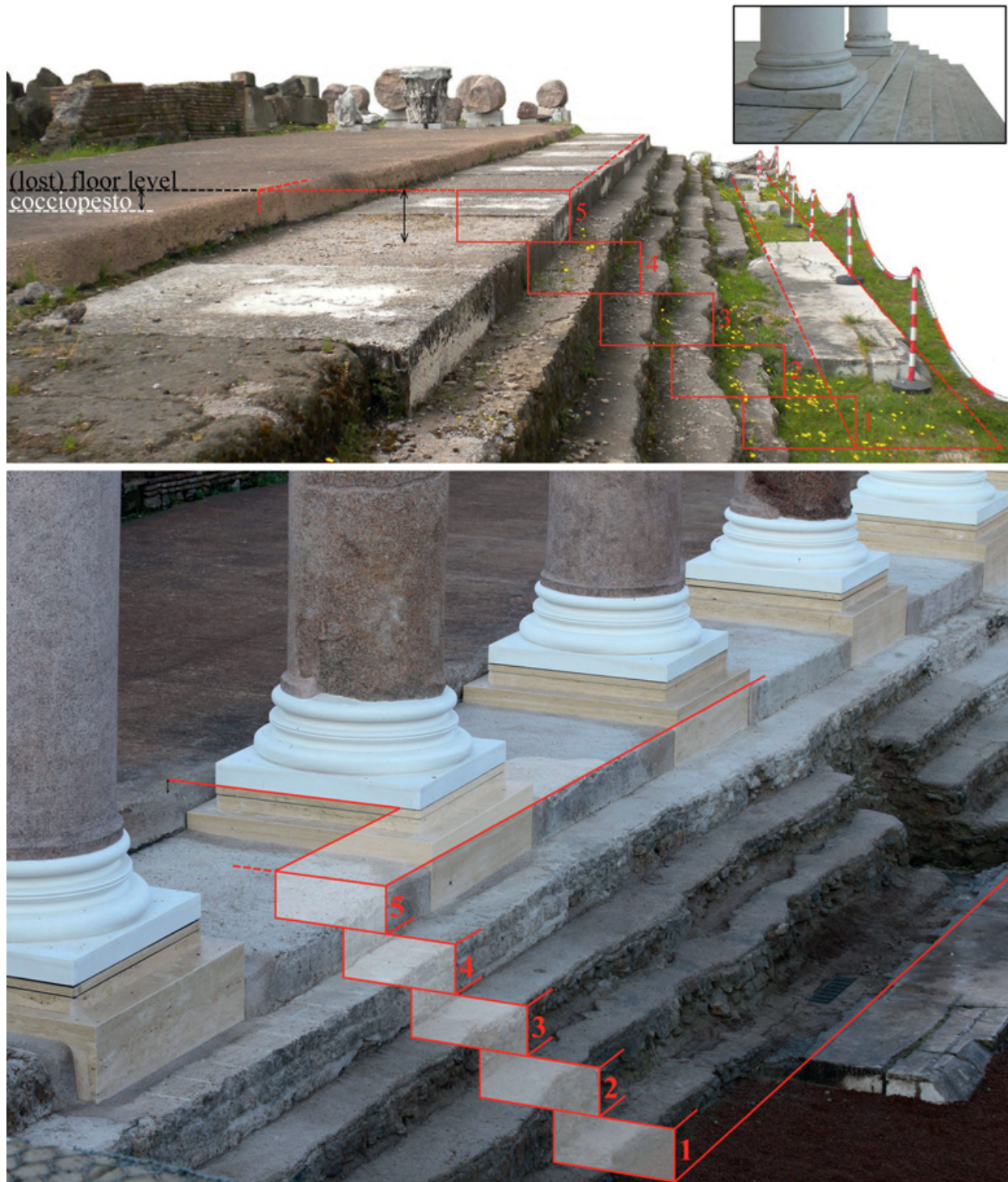
Fig. 13 Author's reconstruction of the five steps of the southwest portico, between the fifth and sixth columns from the Forum of Nerva (top: photos and drawings author; bottom, photo Massimiliano Forconi, drawing author).
