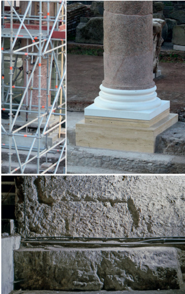
Fig. 16 Top left: column A “inaugurated” on April 21, 2015 (eventually it was dismantled); top right: the same column after reconstruction in December 2015 (photos Massimiliano Forconi). Bottom: trace of the base of a flat pilaster in the Monastery of SS. Cosma e Damiano (photo author).
