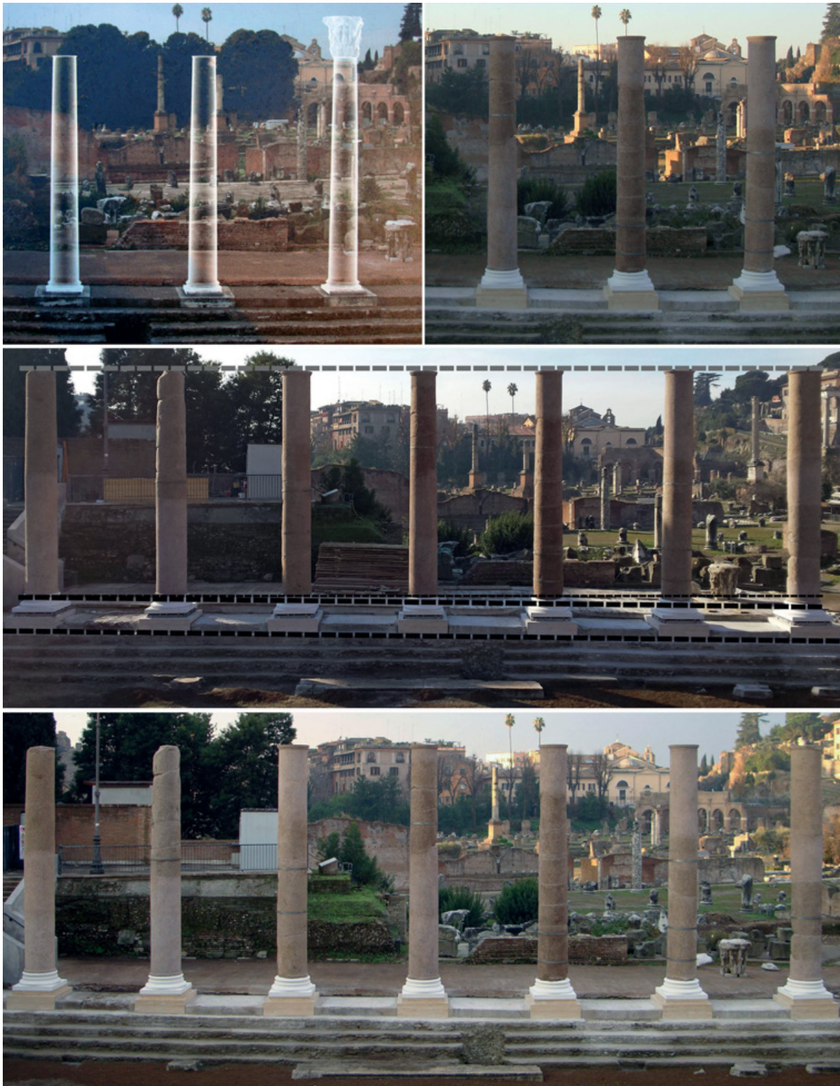
Fig. 15 Top-left corner: reconstruction of three columns (B-C-D) of the southwest portico according to the project by the Sovrintendenza, from the panel displayed just outside the Templum Pacis in 2014 (reconstruction by F. Fabiani for Azimut s.a. s.; photo author). Top-right corner: the same columns after reconstruction (with different plinths) in December 2015 (photo author). Center: the seven columns on December 12, 2015: note the unfinished plinths and the different height of the shafts (photo Paola Tucci). Bottom, the seven columns with finished plinths on December 24, 2015 (photo author).
