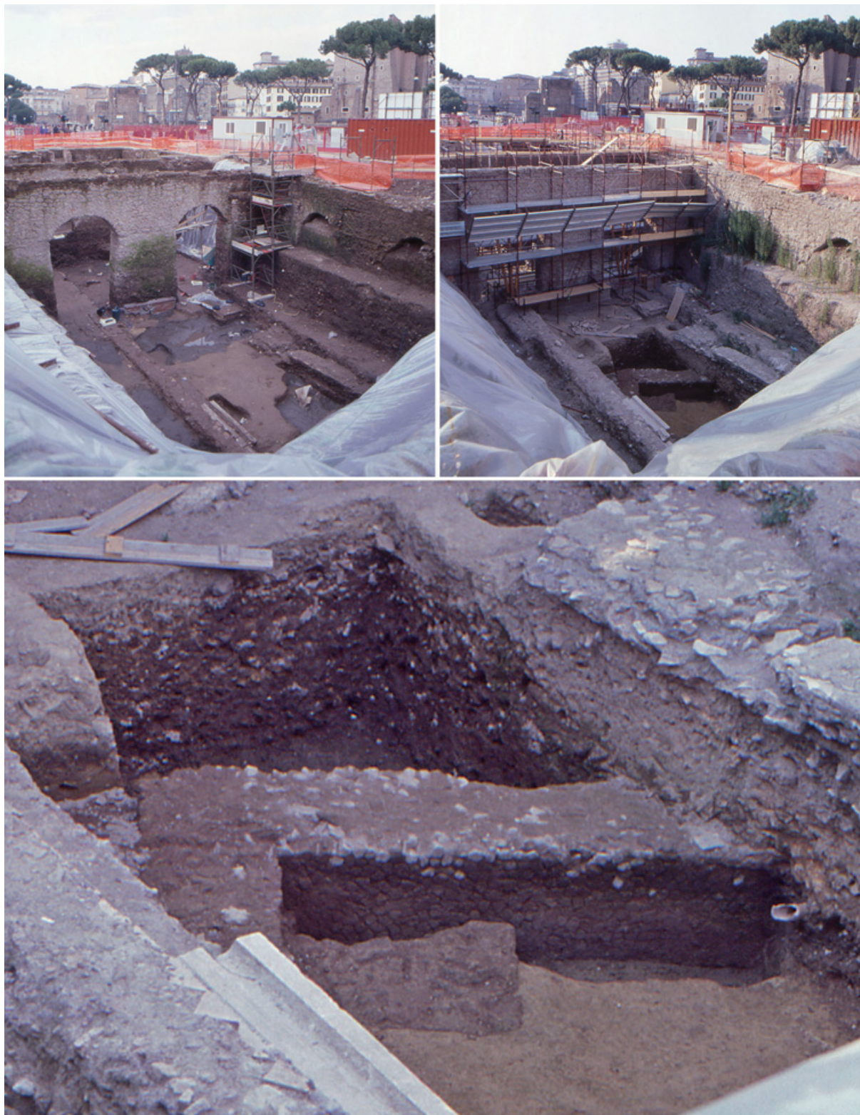
Fig. 5 Excavation of the wall in opus incertum in July 1999 (photos author).
