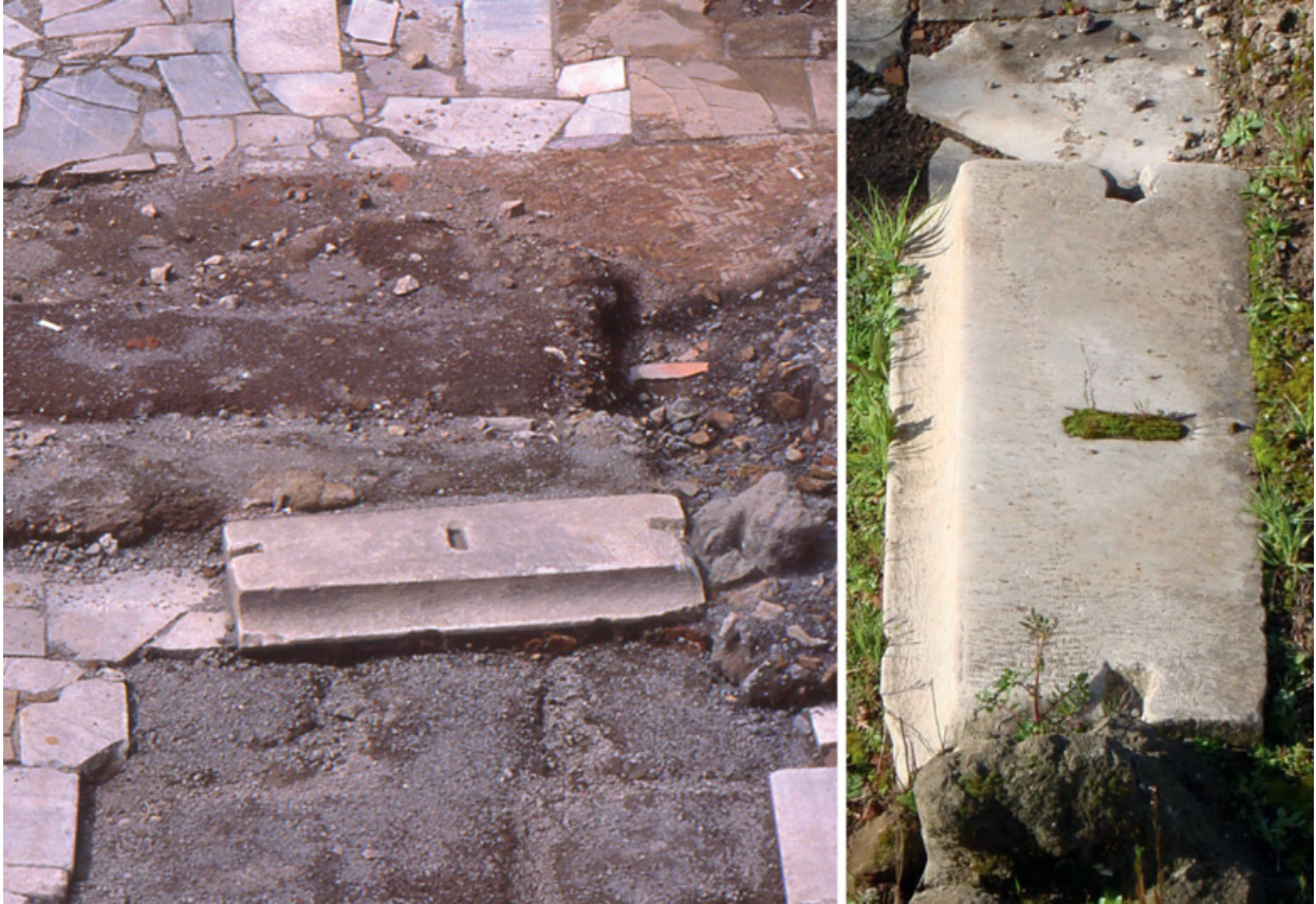
Fig. 24 Marble element attributed to the euripi, but more likely belonging to the attic story (photo author; cfr. Fig. 21, bottom). Note the lewis iron hole and the recesses for metal clamps at both joints.
