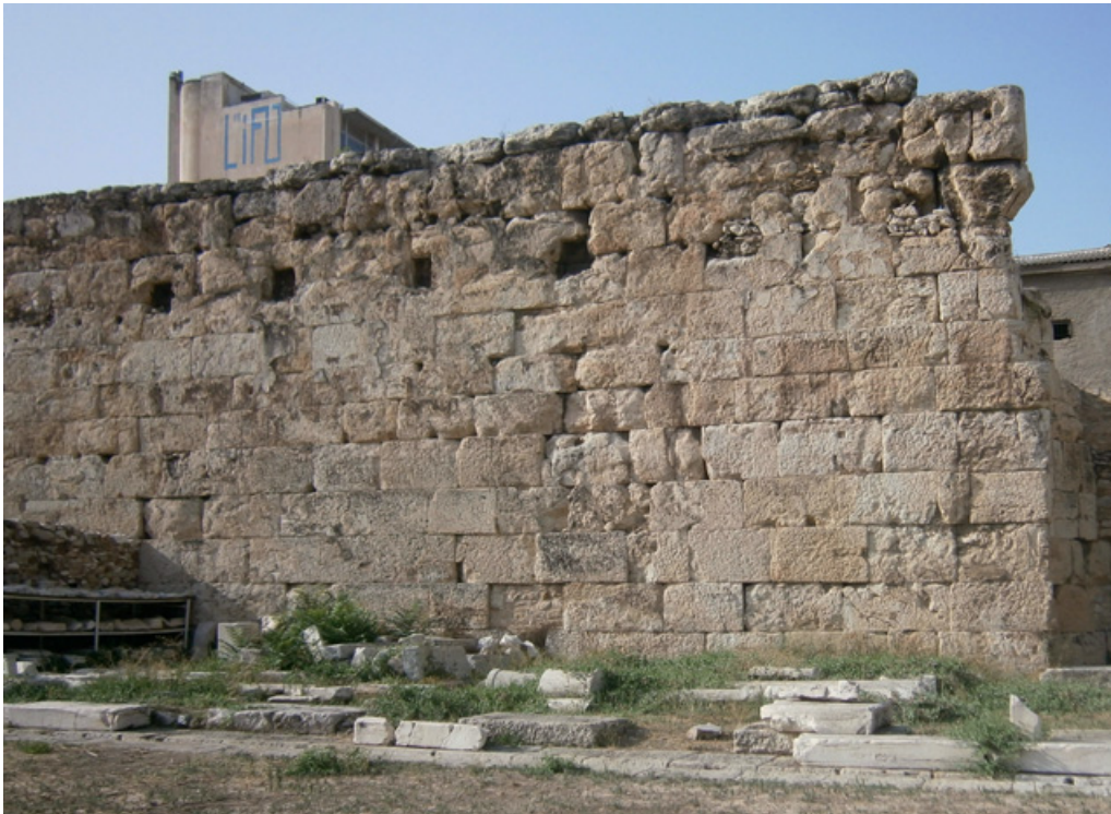
Fig. 35 Rear wall of the left-hand side portico of the Library of Hadrian in Athens, with recesses for horizontal tie beams (photo Laura Garofalo).
