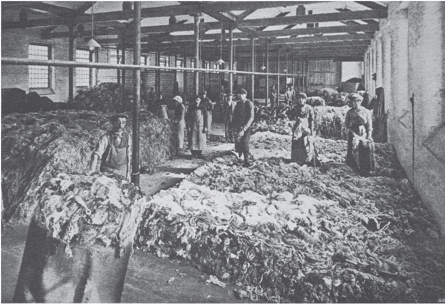
Fig. 1 View of a blending or mixing room at Redmayne and Isherwood Ltd., Kirkham, manufacturers of cotton and engine waste.
