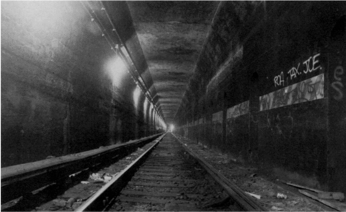
Figure 1.4 A subway tunnel beneath Chinatown
