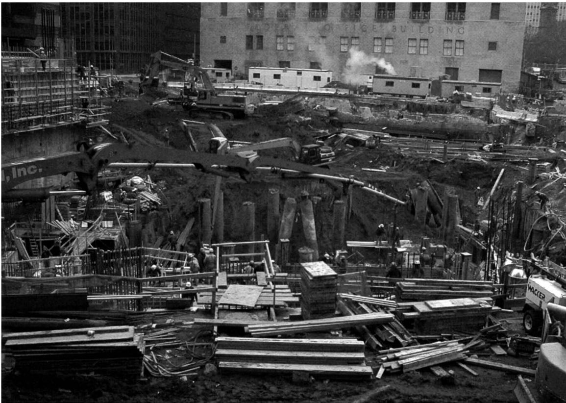
Figure 2.5 Rebuilding the foundation of 7 World Trade Center in 2003
