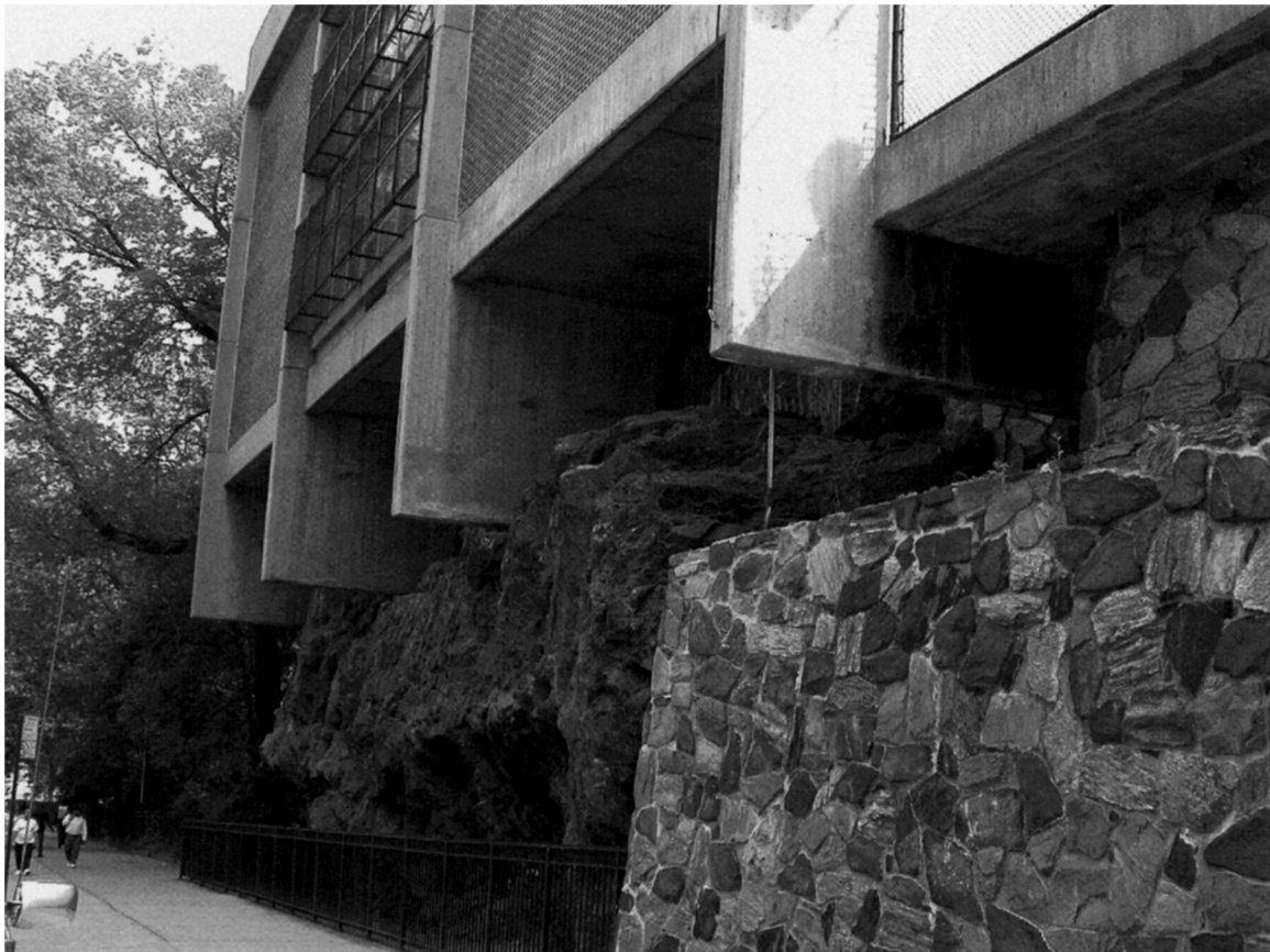
Figure 2.3 These building supports on West 123rd Street rest on bedrock above street level
