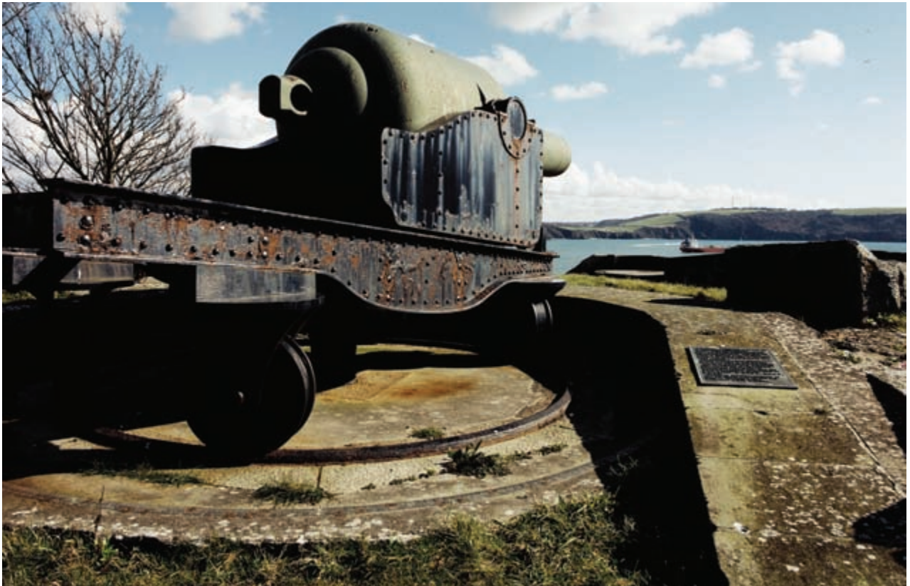
Plate 6 Drake's Island, Plymouth. 12in RML on reproduction mounting on emplacement no.5 of the upper battery. On the skyline in the distance is Fort Staddon. (© Crown Copyright. NMR, AA98 01876)
