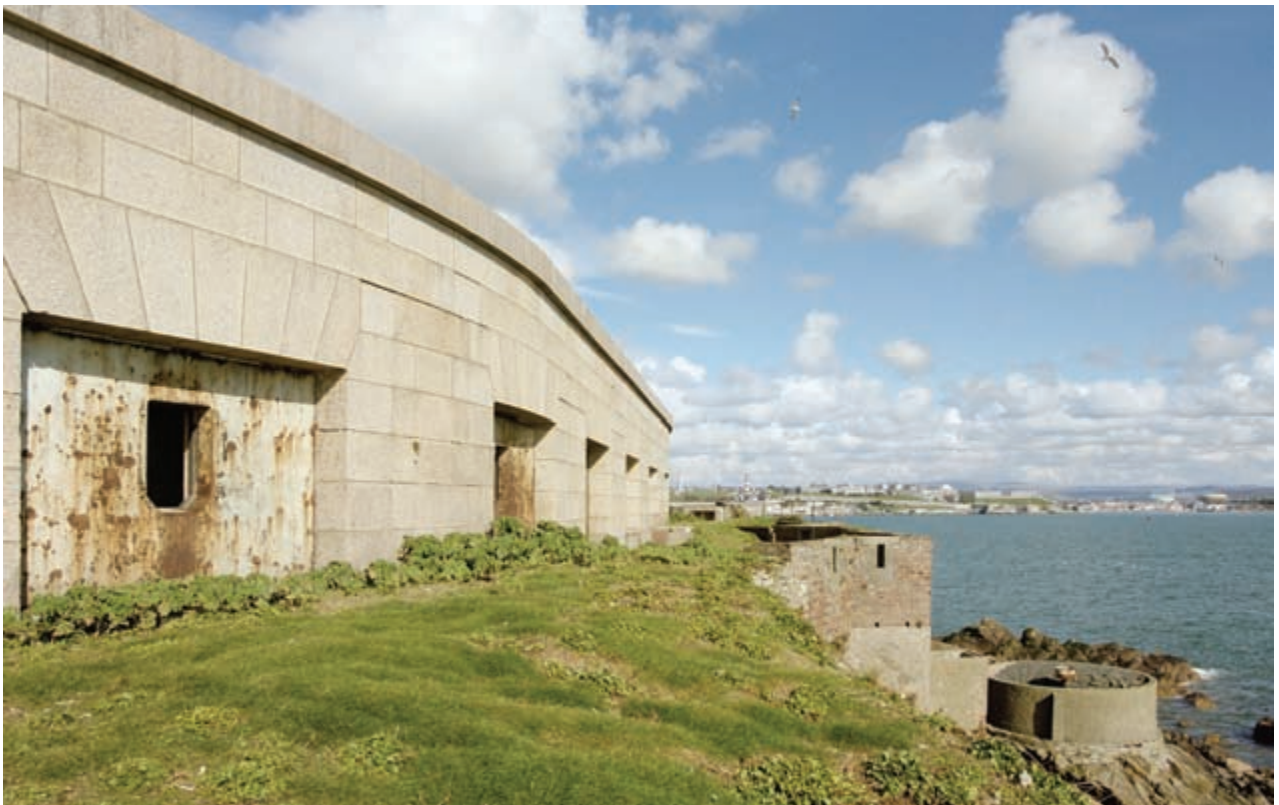
Plate 7 Drake's Island, Plymouth. Seaward face of casemate battery, showing granite construction and iron shields. Plymouth Hoe and de Gomme's Royal Citadel can be seen in the distance. (© Crown Copyright. NMR, AA96 02250)
