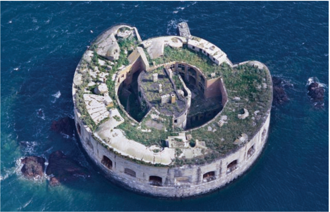
Plate 9 Stack Rock Fort, Milford Haven, from the air looking north. The original small fort of 1852 can be seen in the centre, surrounded by the 1860s casemated battery. (© Crown Copyright: RCAHMW 2002-cs-0770)
