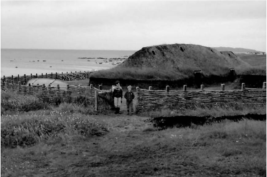
1.2 Replica of Viking buildings in L'Anse aux Meadows, Newfoundland. Constructed of sod over a timber frame ca. AD 1000, they form the only authenticated Viking settlement in North America. G. Bassler photo, 1985.
