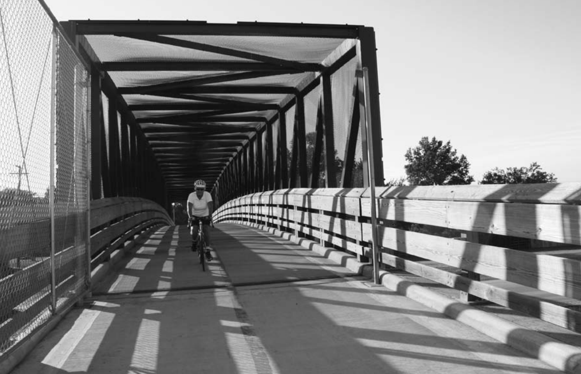
Bicycle/pedestrian bridge over US 24
