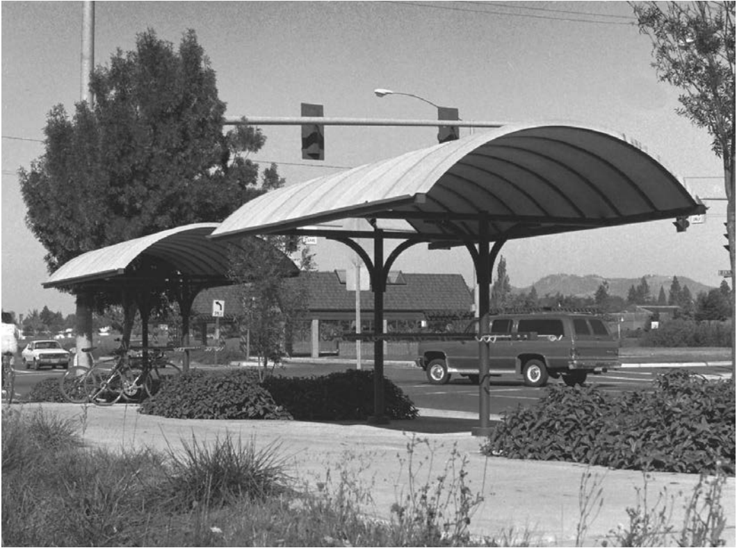
3. Lane Transit District Bicycle Shed, Eugene, Oregon, 1984. Far from being an undistinguished shed, the bicycle cover here is part of a citywide network of shelters designed to encourage the use of bus transportation. Photo: L. M. Roth.
