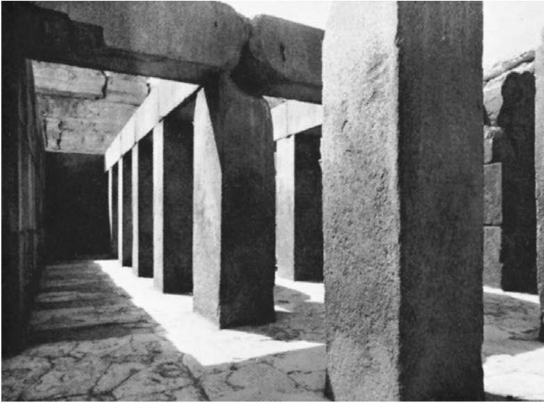
3.11. Valley Temple, Pyramid of Khafre, Giza, Egypt, c. 2570–2500 BCE. This is one of the purest and most direct expressions of stone post and lintel construction. Photo: Hirmer Verlag, Munich.
