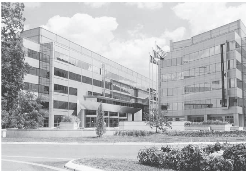
PHOTO 2.3 NRO headquarters, Chantilly, Virginia. Photo credit: NRO.
