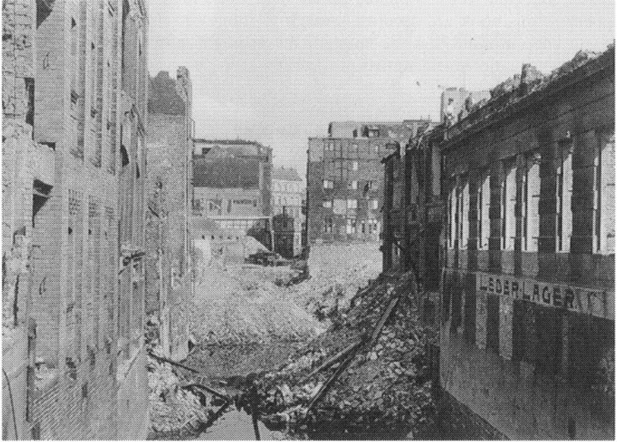
Hamburg, rubble in the Catharinenstraße canal. The city disposed of much of the rubble by filling in many canals, including this one. (Source: Staatliche Landesbildstelle Hamburg, 6564.)
