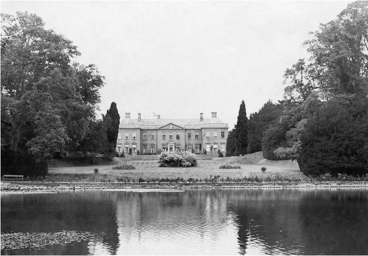
Figure 1.1. Holme Lacy, the Scudamore manor house in Herefordshire, England, as shown c. 1890.
