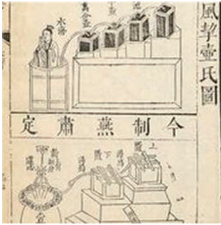
Figure 17 Lu Cai's inflow type clepsydra with are three compensation tanks. (top) Yan Su's inflow type clepsydra, has an overflow tank on the ground. (bottom) Illustration from Liu Jing Tu Kao 六經圖考 of Yang Jia (c.1110–84), reprinted in 1722, Book vi 37.
