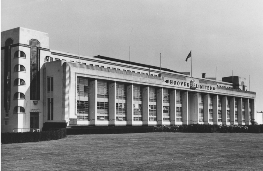
Plate 1.1. Egyptianizing, Art-Deco, Modernistic former Hoover factory, Western Avenue, London (1931–8), by Wallis, Gilbert, & Partners: the long front, with battered sides, is a version of an Egyptian temple-front, whilst loculi -like openings are recalled in the windows of the towers (which also sport tall windows with heads composed of the chamfered or canted pseudo-arch)
