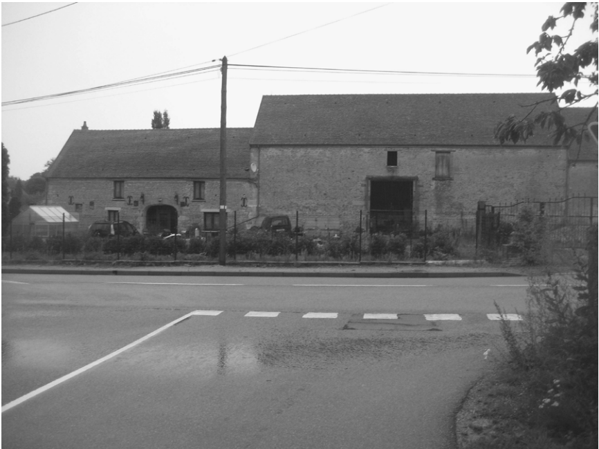
Figure 1.1 The site and remains of the Viennes' home in Nonant.
