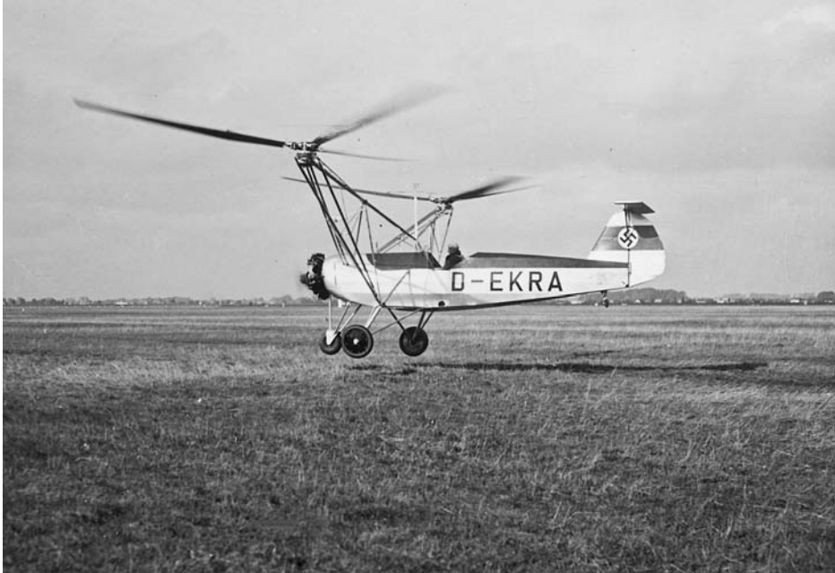
Fig. 1.1 The Focke-Wulf Fw-61 was the first helicopter to move beyond the experimental stage and was capable of extended flights. The hull was based on that of an Fw Stieglitz aeroplane. Note the vestigial airscrew that simply cools the engine. (Steve Coates)
